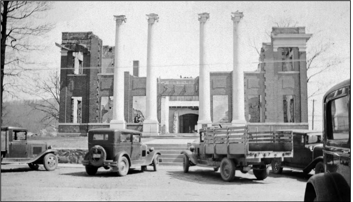
Alleghany County Courthouse after the 1933 fire that caused an estimated $18,000 in damages to the town of Sparta. County records were rescued, however, and are a rich resource available to researchers, today. This rare photo shows the building after cleanup and ready for reconstruction. Thanks to Hugh W. Halsey for allowing us to publish it here.
