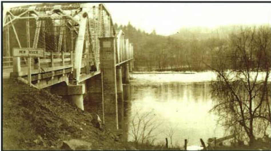
The old US21-221 bridge over New River- part of the Lakes-to-Florida Highway.
